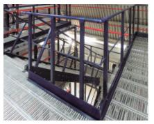
Railings. Protective rails are built with round and rectangular tubes that are joined together. Protective skirting is fitted to its base to prevent objects falling from the mezzanine floor.
