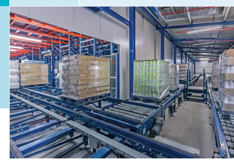
Conveyor systems represent an ideal combination between the efficiency of the stacker cranes and the entry, dispatch and handling processes of the load units. Logistics operations require a continuous flow of materials, as pallets and/or boxes must be taken from a storage or production location or from an overflow warehouse to dispatch or production areas.
