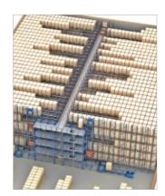
**Automatic Pallet Shuttle** installation with transfer car A gangway type structure is installed that allows the movement of a transfer car on each level, whose task is to carry out movements from the lifts to the storage channels of each level. Thus, the number of movements or cycles/hour is multiplied by the number of levels in a warehouse, combining high capacity with a large number of movements.
