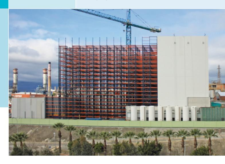
The clad-rack warehouse is the ideal solution for stacking goods high, as its design ensures the racking structure forms a compact unit along with the roofing and the cladded walls of the warehouse, removing the need for building work.
