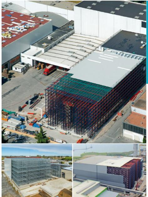
Clad-rack warehouses can use either automated systems or pallet racking, drive-in and cantilever racking, or the Pallet Shuttle, etc.
