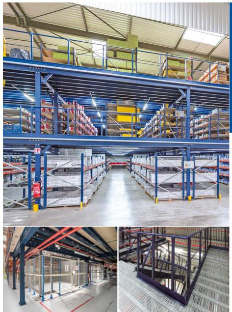
Mezzanine floors can be completely disassembled and reused.
